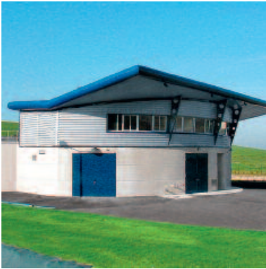
STATION D'ÉPURATION AUTONOME
